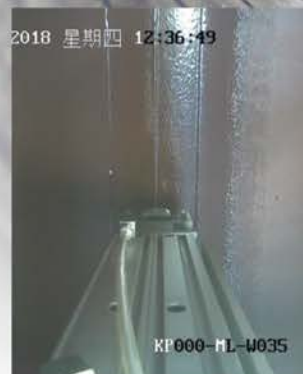
Applied Internal Field Joint Coating on Weld
